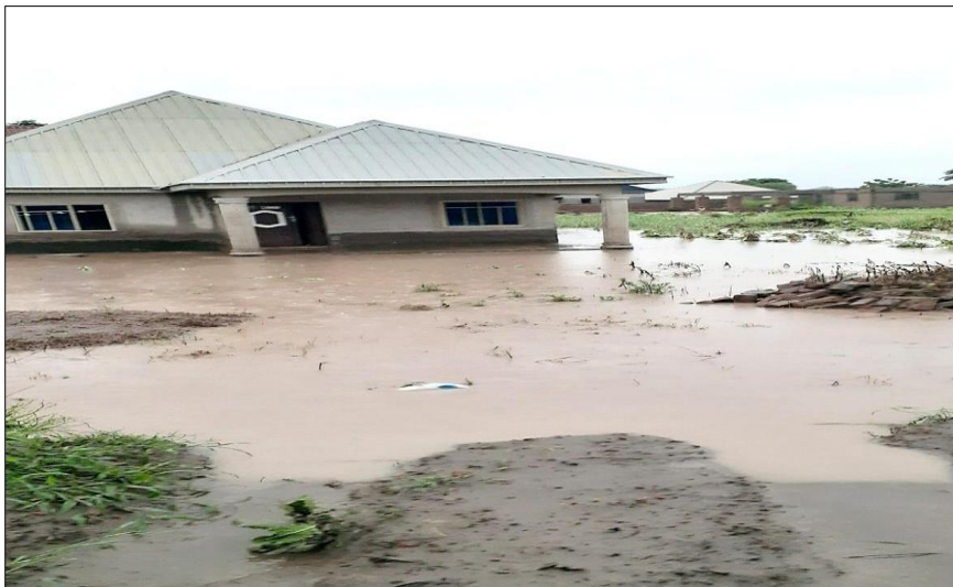
Fig. 6. Flooded buildings in the wetland area in Ugondo Layout Makurdi.
