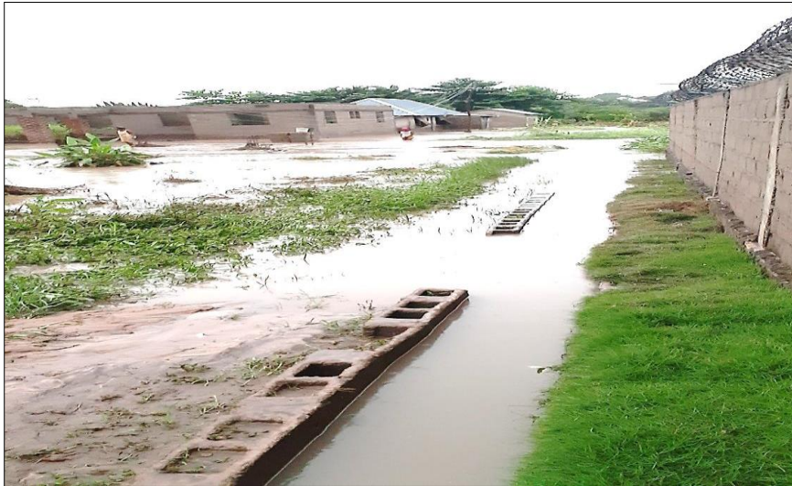
Fig. 5. Flooded buildings in wetland area in Ugondo Layout Makurdi.
